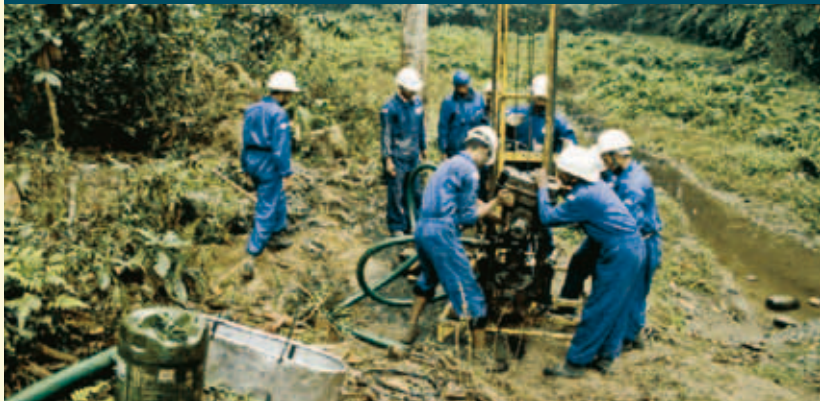
Asian Oilfield crew conducting shot hole drilling with mechanized drilling rig
