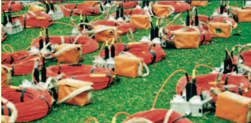
Aram Aires equipment and cables laid out at a project site
