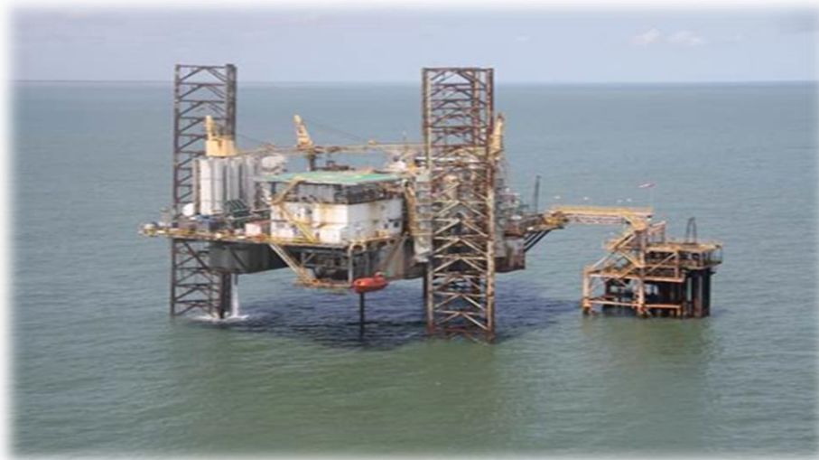
Nigeria (Upgrade existing offshore MOPU)
