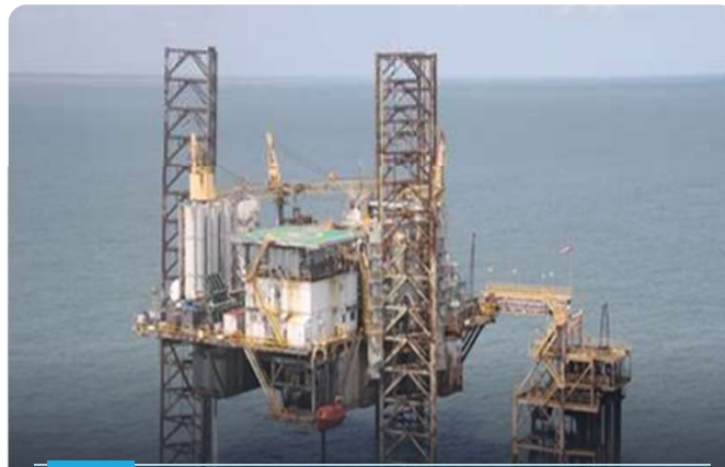
Nigeria, (Upgrade existing offshore MOPU)
